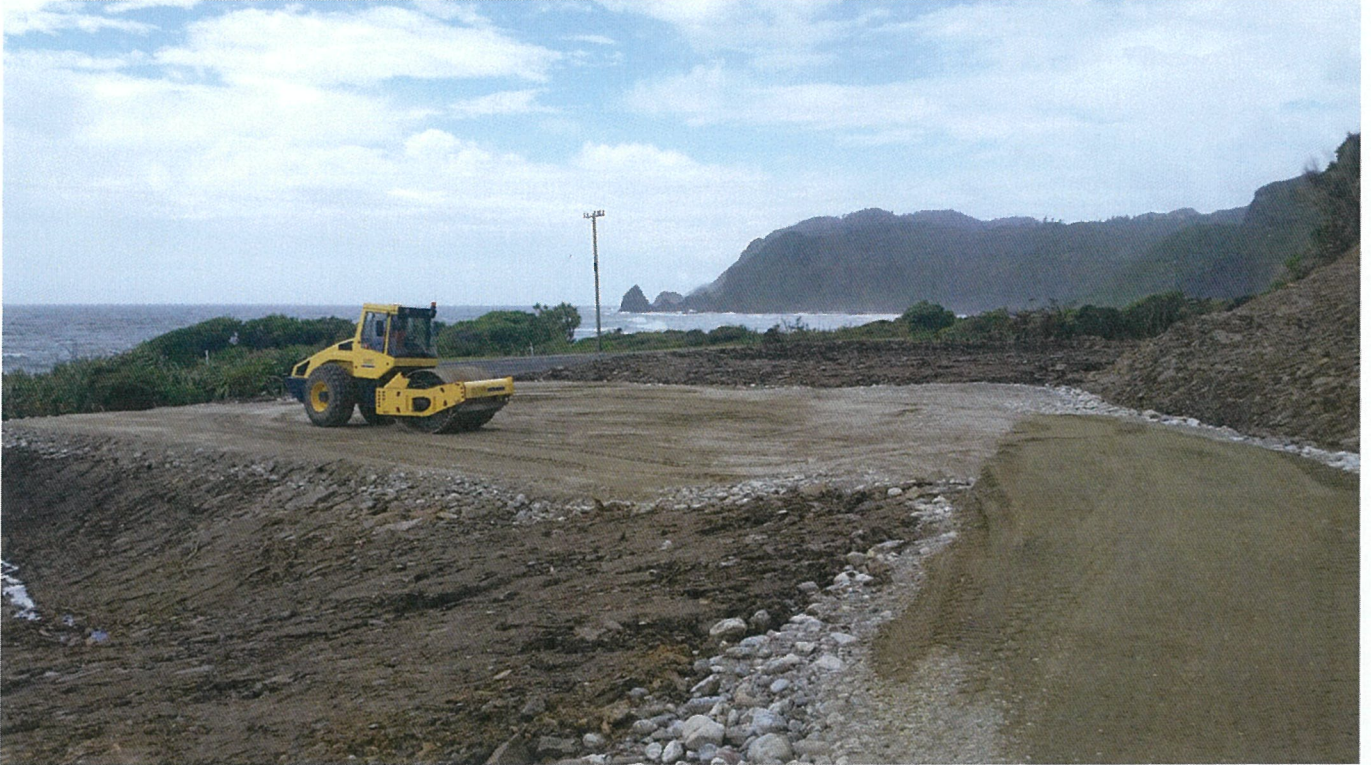
Whitehorse site. Building pad at north end.
