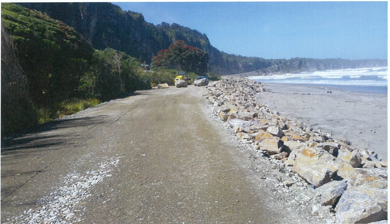
Looking south along completed seawall extension
